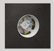
Rinse pipes using a preassembled flushing device.
